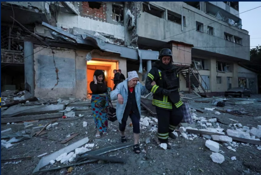
Evacuation from an apartment building damaged by a Russian drone strike, Kharkiv, Ukraine, 12 June, 2025. Credit: Vyacheslav Madiyevskyy / Reuters
